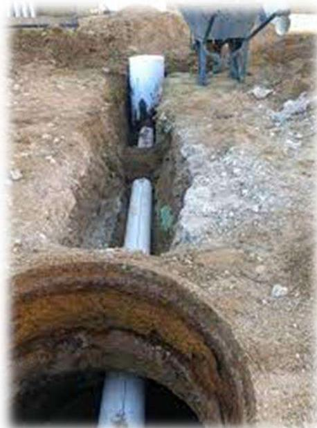
Sewage is dealt with at Al-Nahrain University by draining this water through large underground pipes and connecting them with the public sewage pipes that were prepared by the Capital Municipality.
